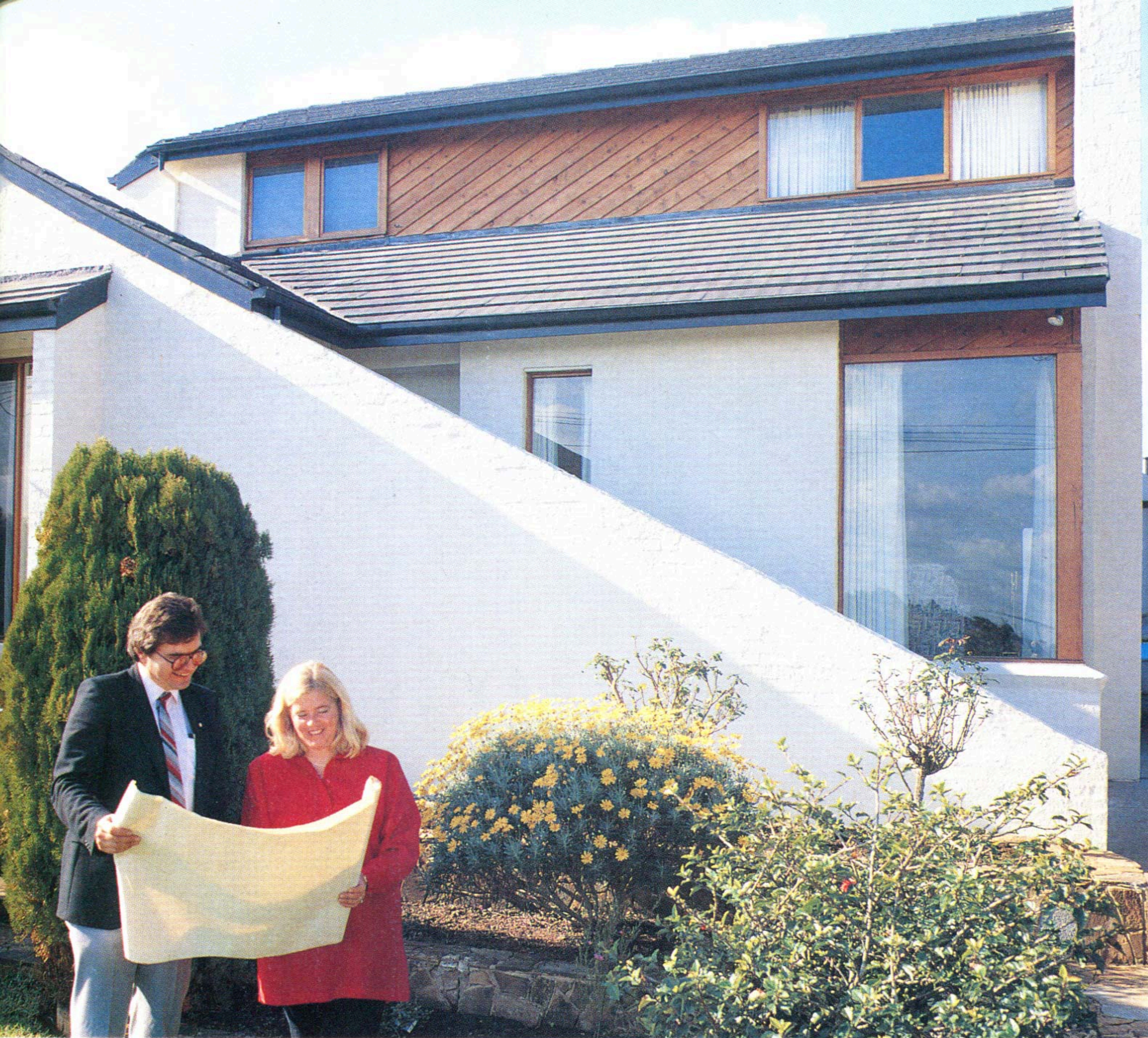
Above: The house as it was (opposite) and, as it is today. Owner Janine Clark and architect Andrew Fedorowicz study the plans. The old hipped roof has gone but the slope and the left peak remain the same. The roof's overhang and the extended "boxed" walls of the bedroom window and the diagonal wall give protection from the sun in summer. Left: The winter sun warms the family room and the Clarks rarely use the ducted heating. The table is of 140-year-old oregon from the old Newmarket saleyards.
